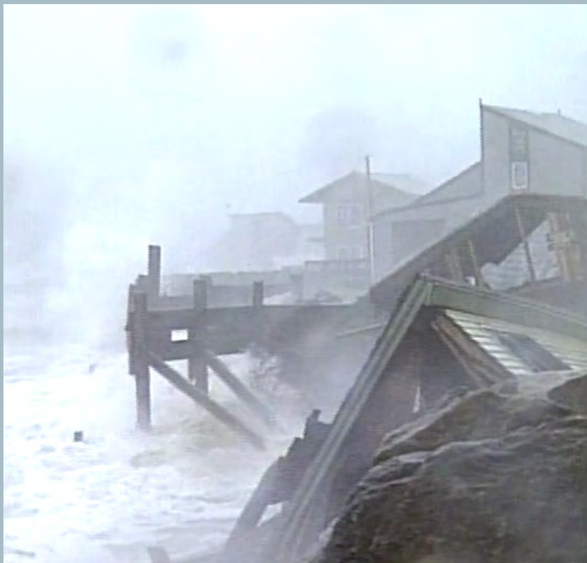
Damage in Maine from Hurricane Bob in 1991, the last Category 2 hurricane to make landfall on Maine's coast. © WGME
